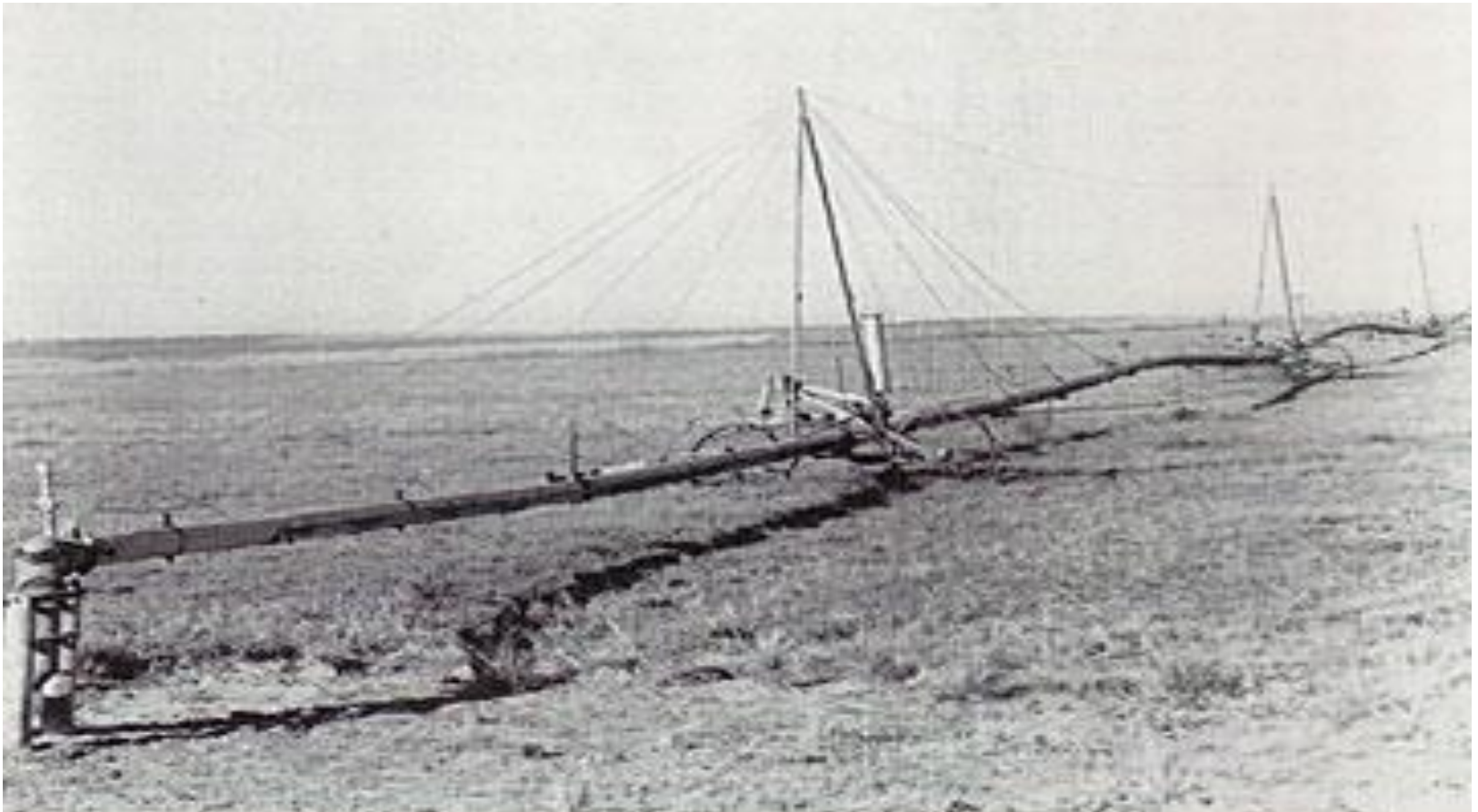
Frank Zybach's first center-pivot irrigation system, near Strasburg, Colorado. He started with a low pipe that was later raised to run over corn fields. UNL.
